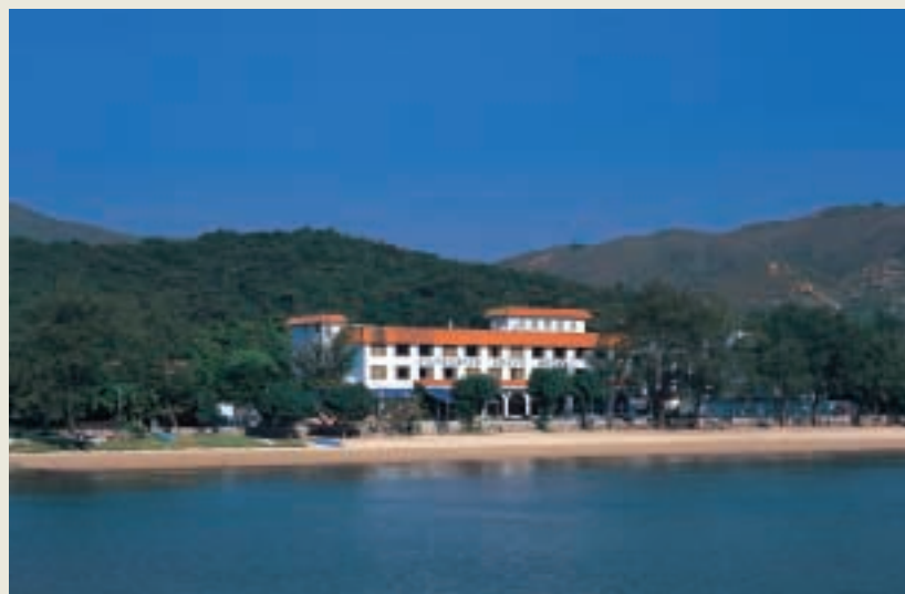
Silvermine Beach Hotel has benefitted from its location close to the newly-opened Asia World Expo.
